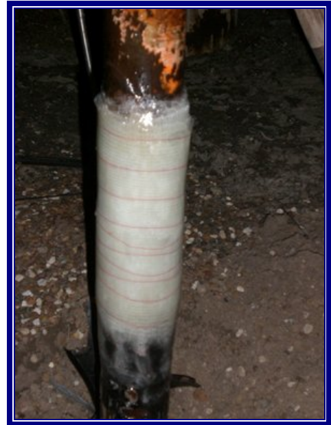
After; Corrosion Contained and Repaired
